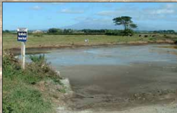
Unlined pit for synthetic based drilling mud at BTW Brown Road landfarm, Taranaki, TRC doc 987702, 2012.
