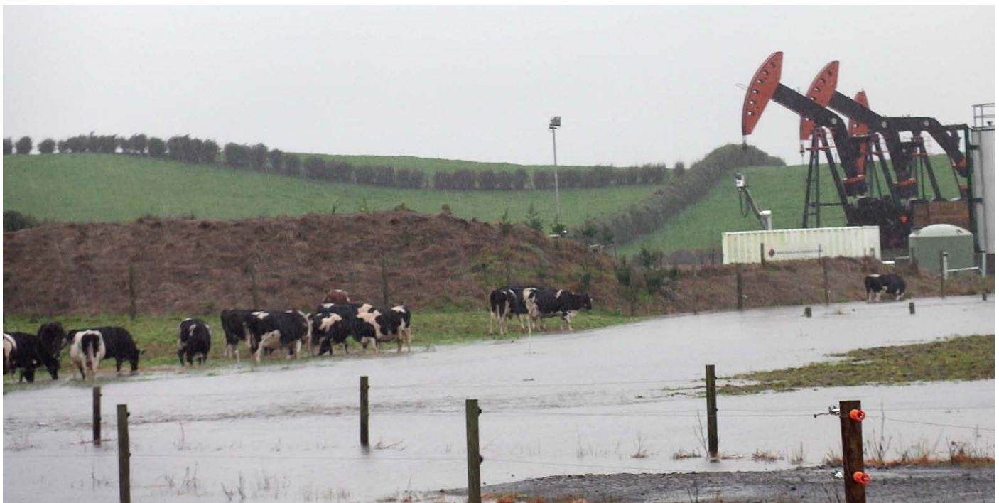
Figure 6. Copper Moki wellsite during rainstorm
