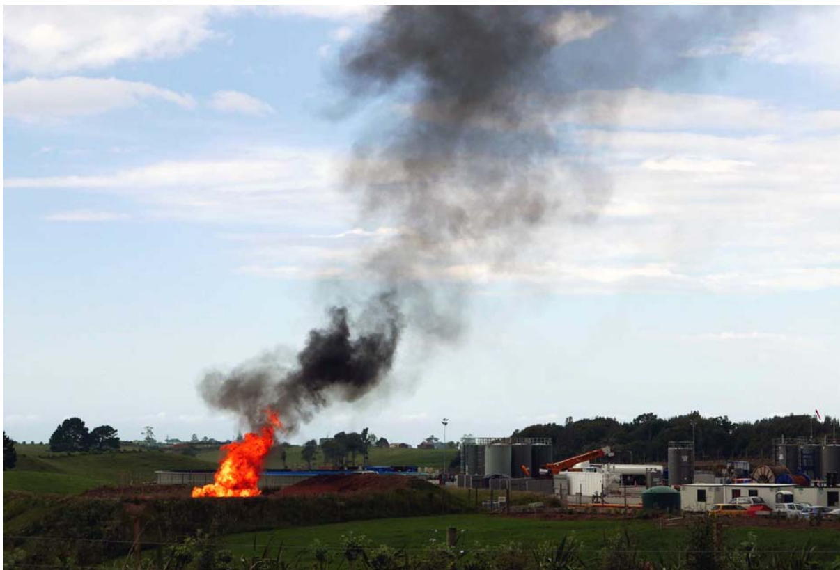
Figure 8. Smoky flare at Todd Energy Mangahewa-E Wellsite on 29 December 2014, Tikorangi
