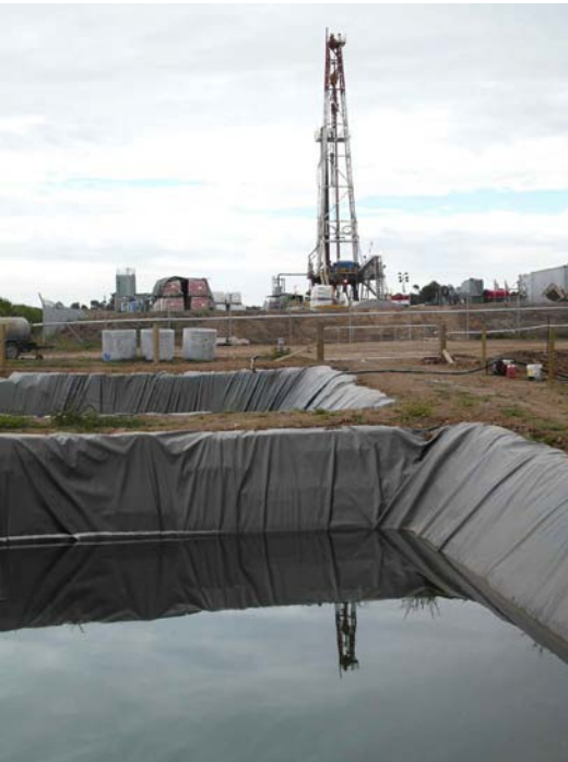
Mangahewa-C wellsite. Photo by Fiona Clark, 11 April 2013.
