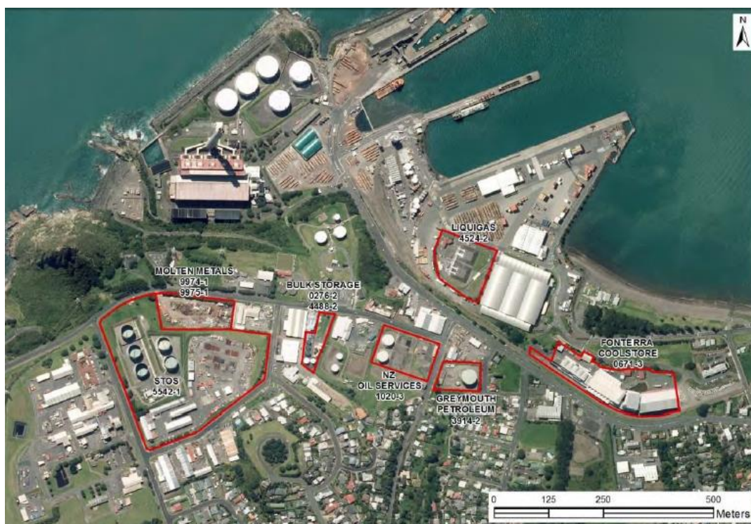
Paritutu Tank Farm and consent holder property boundaries in the Hongihongi catchment (TRC, Feb 2016)
