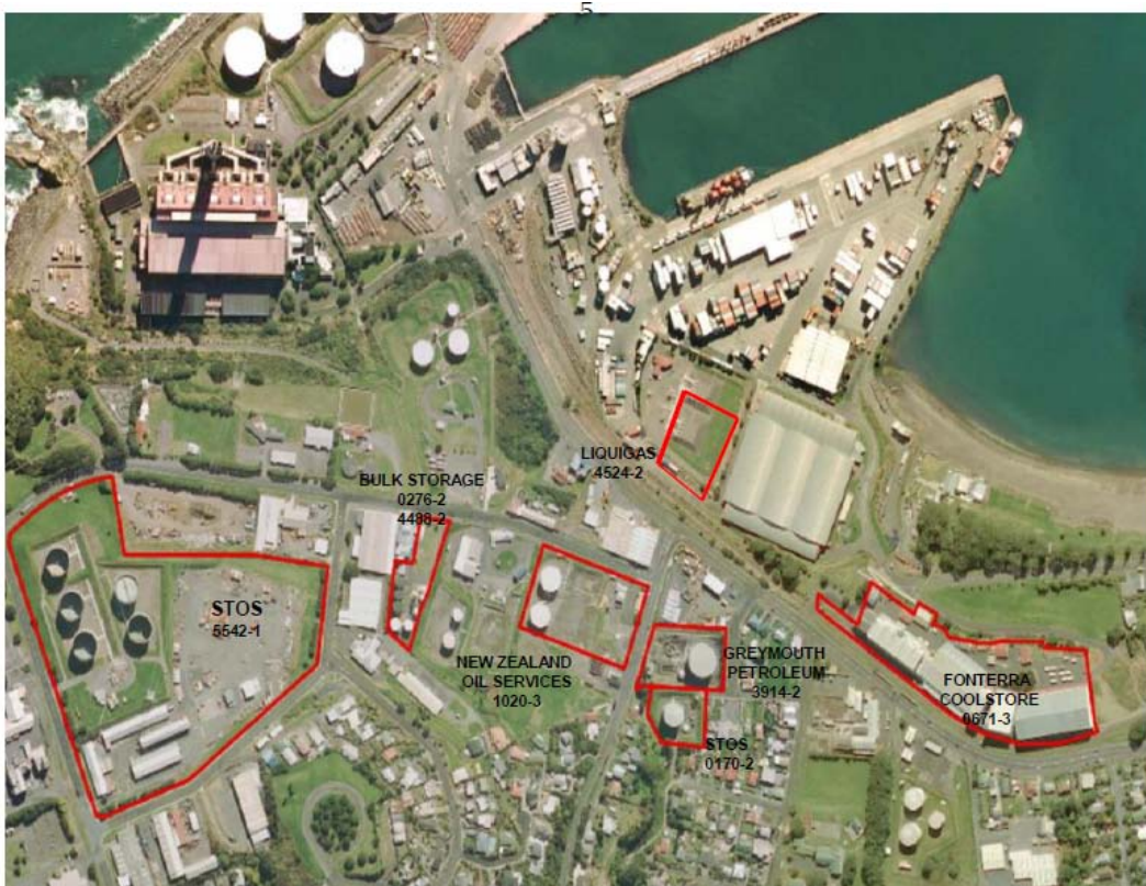
Paritutu Tank Farm and consent holder property boundaries in the Hongihongi catchment (TRC, Oct 2014)
