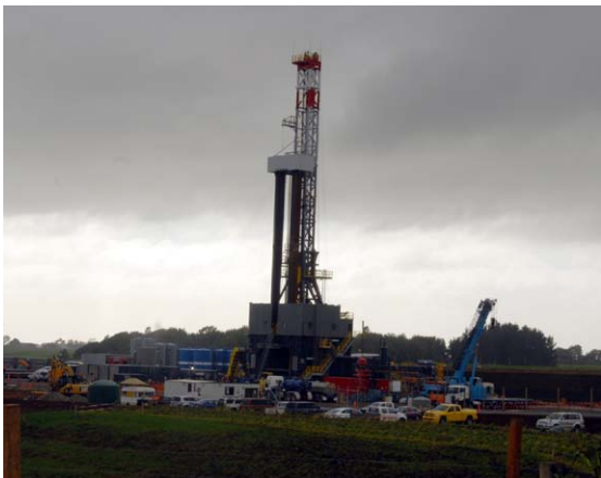
Todd Energy Mangahewa-E wellsite, 2014.
